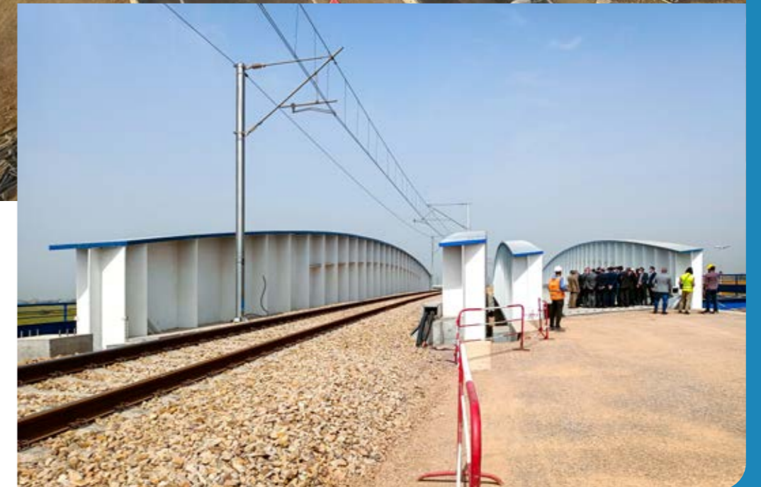
“ The two new metal bridges of the rail service from Mohammed V airport to PK 12 of Casablanca - Berrechid highway
